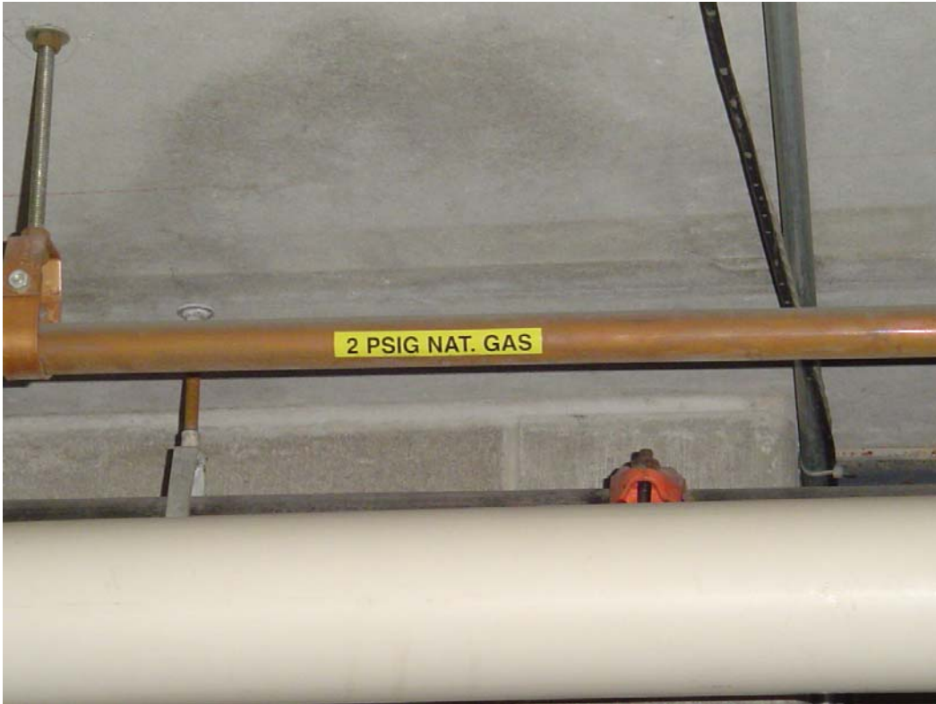
Typical Natural gas distribution piping
