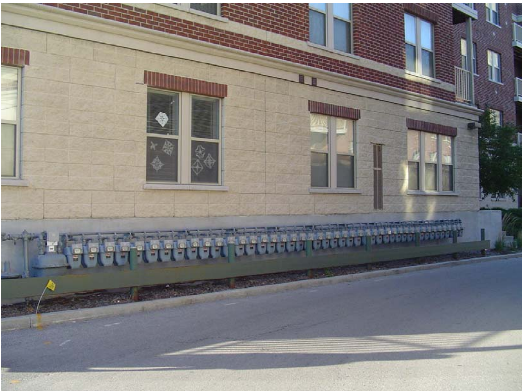
Gas meters and manifold
