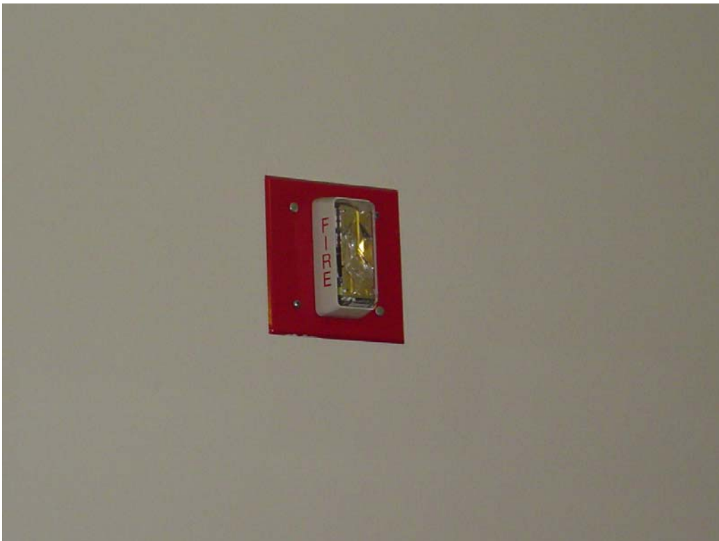
Typical Fire Alarm System Audible Visual Alarm Device
