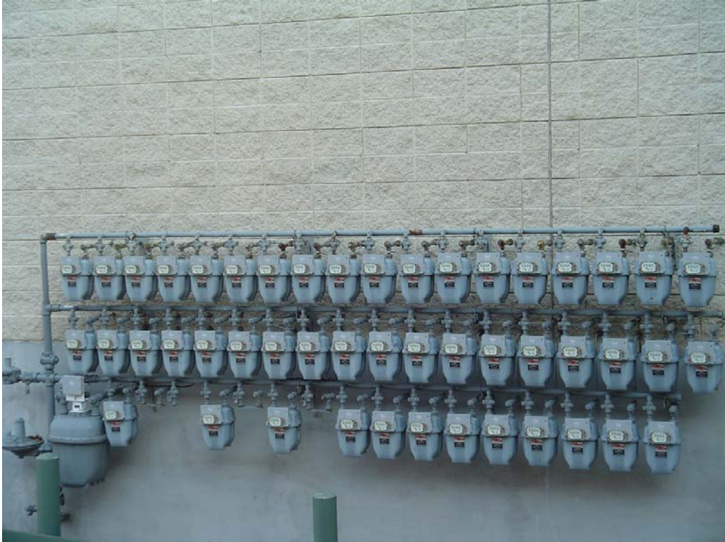
Gas meters and manifold
