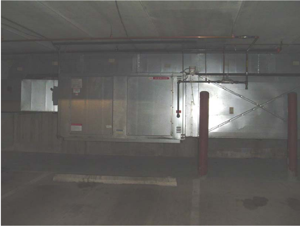
Building “B” Make up air unit
