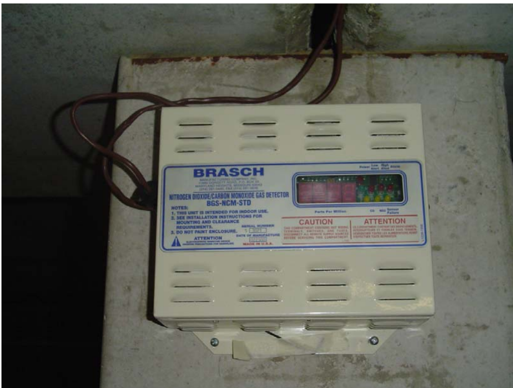
Nitrogen Dioxide / Carbon Monoxide Sensor
