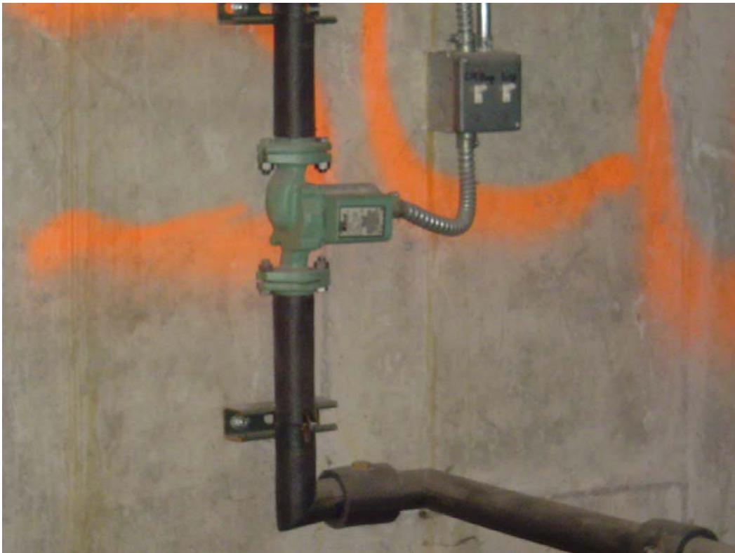
Building “B” hot water circulation pump
