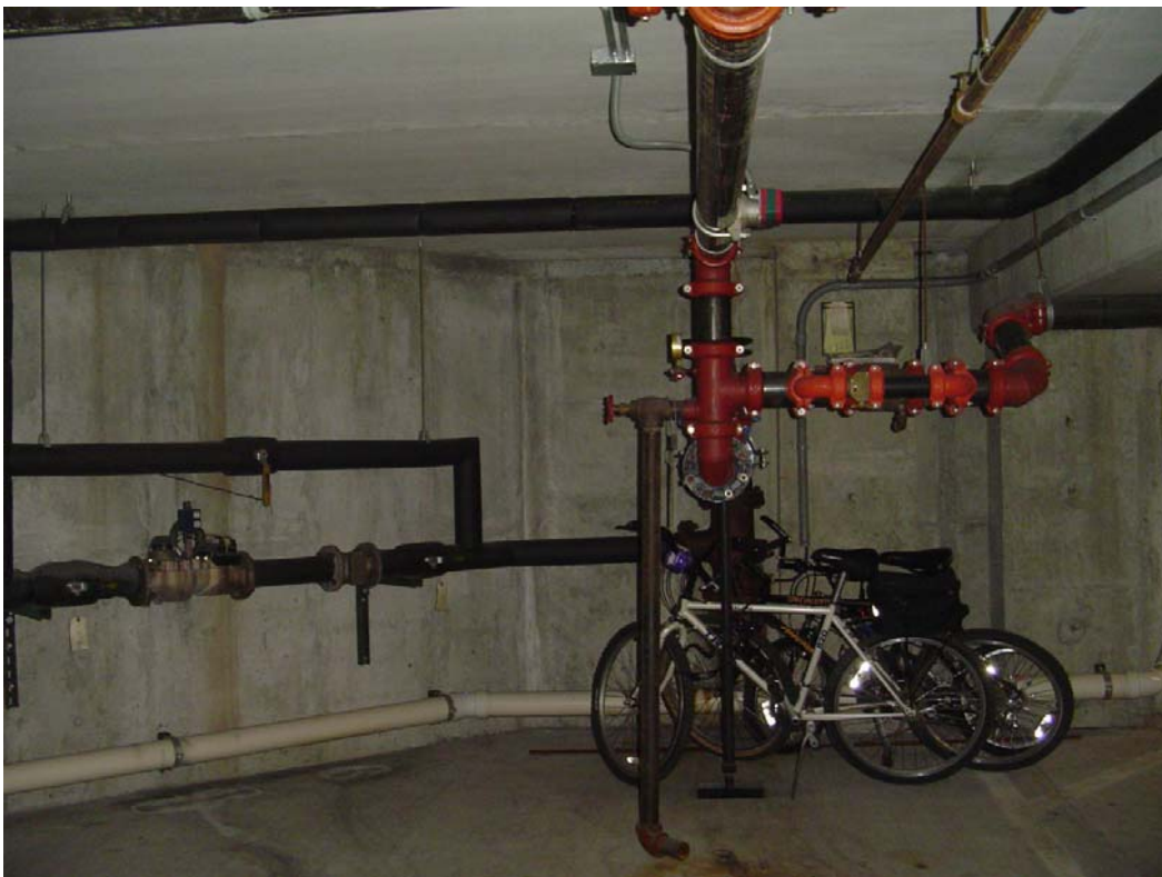
Water main, Fire protection back flow device
