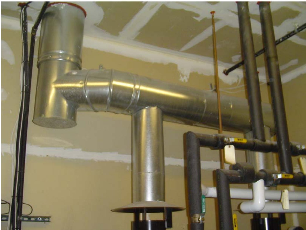
Building "A" Water heater venting
