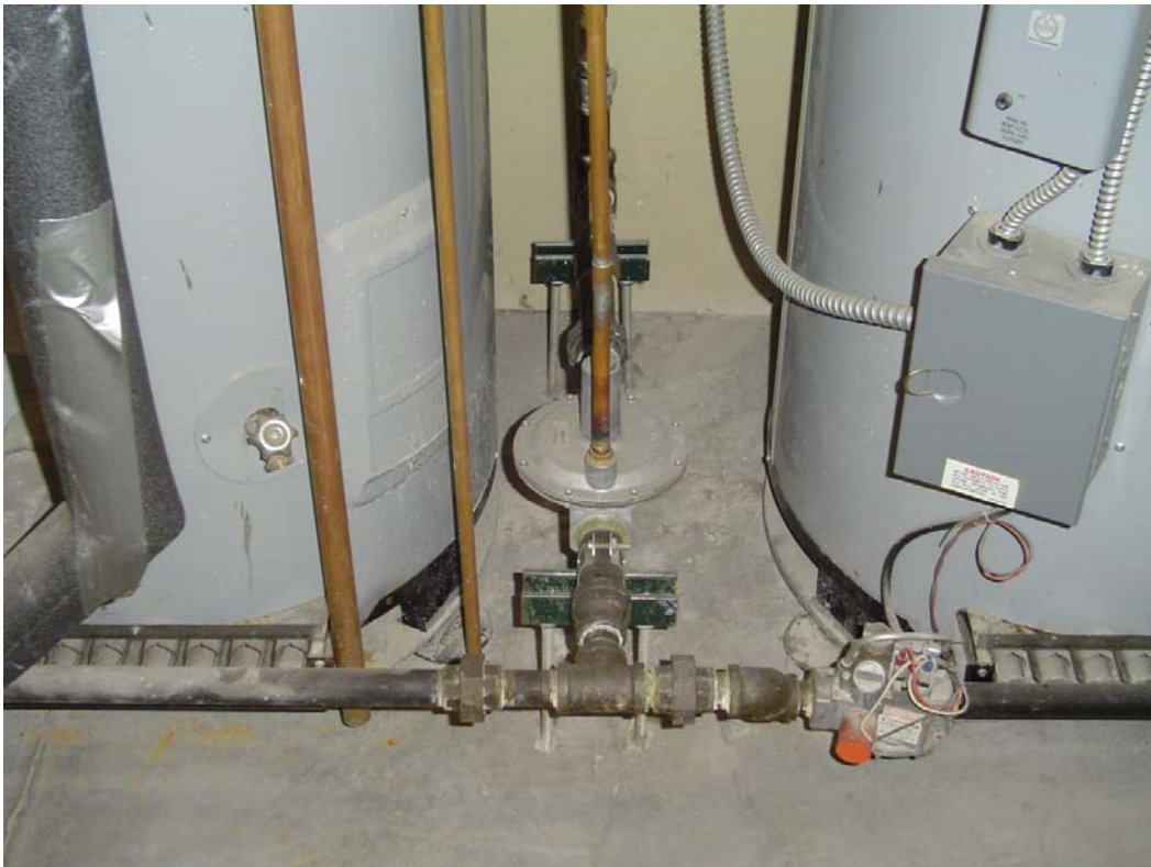
Water heater natural gas connection
