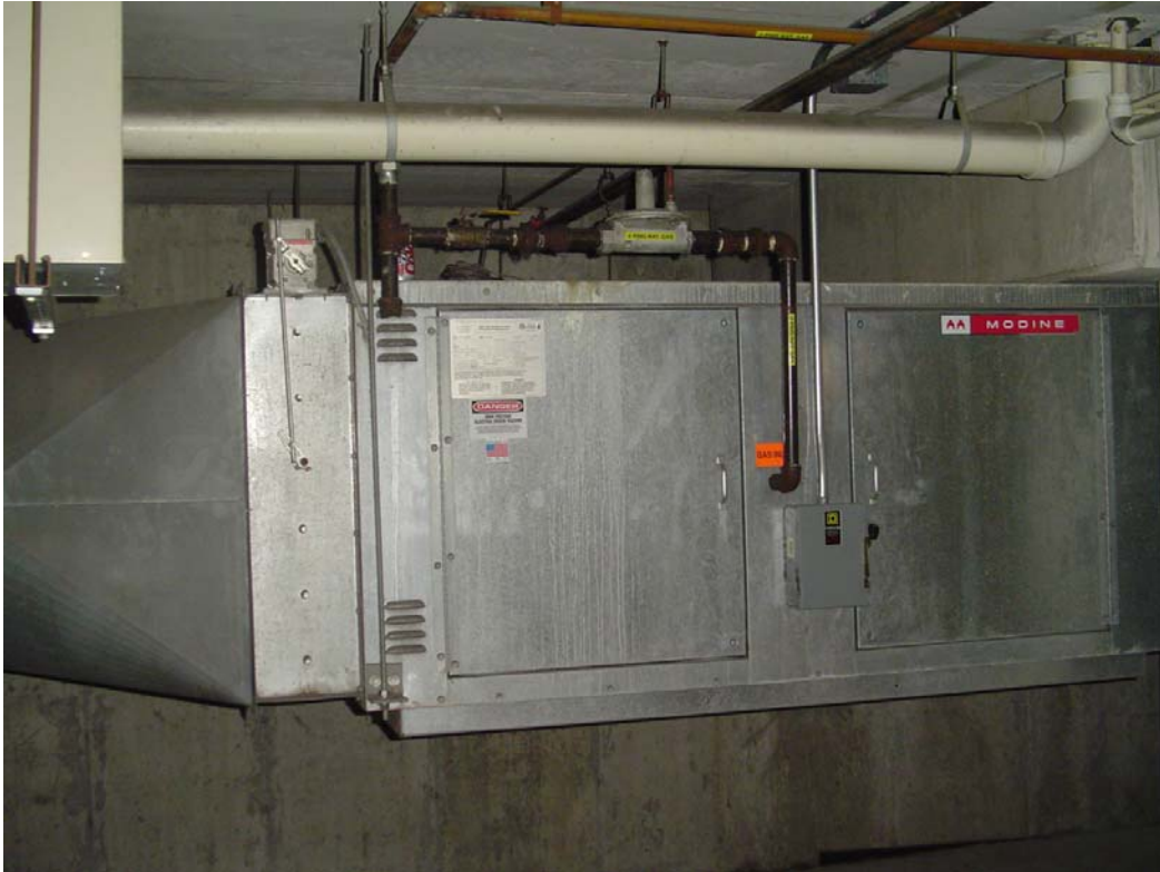
Building “A” Make up air unit.
