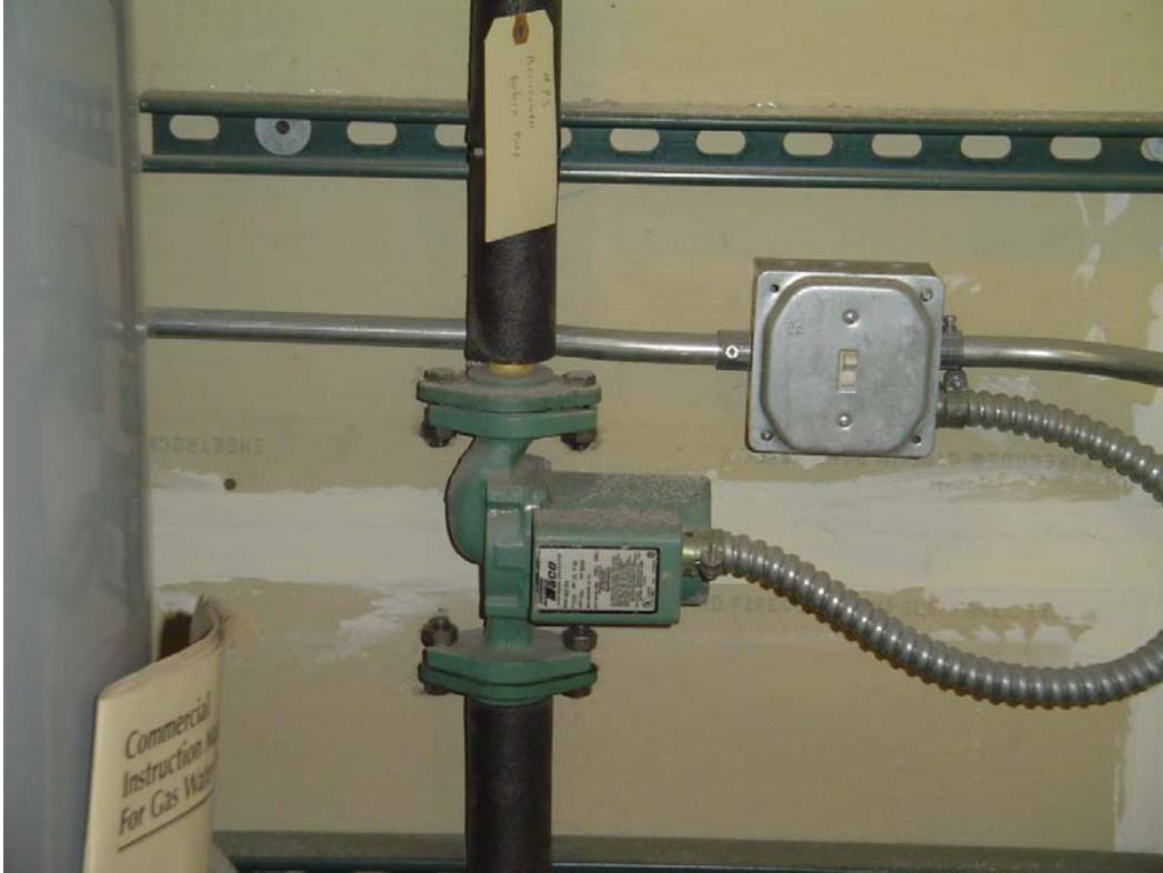
Hot water circulating pump
