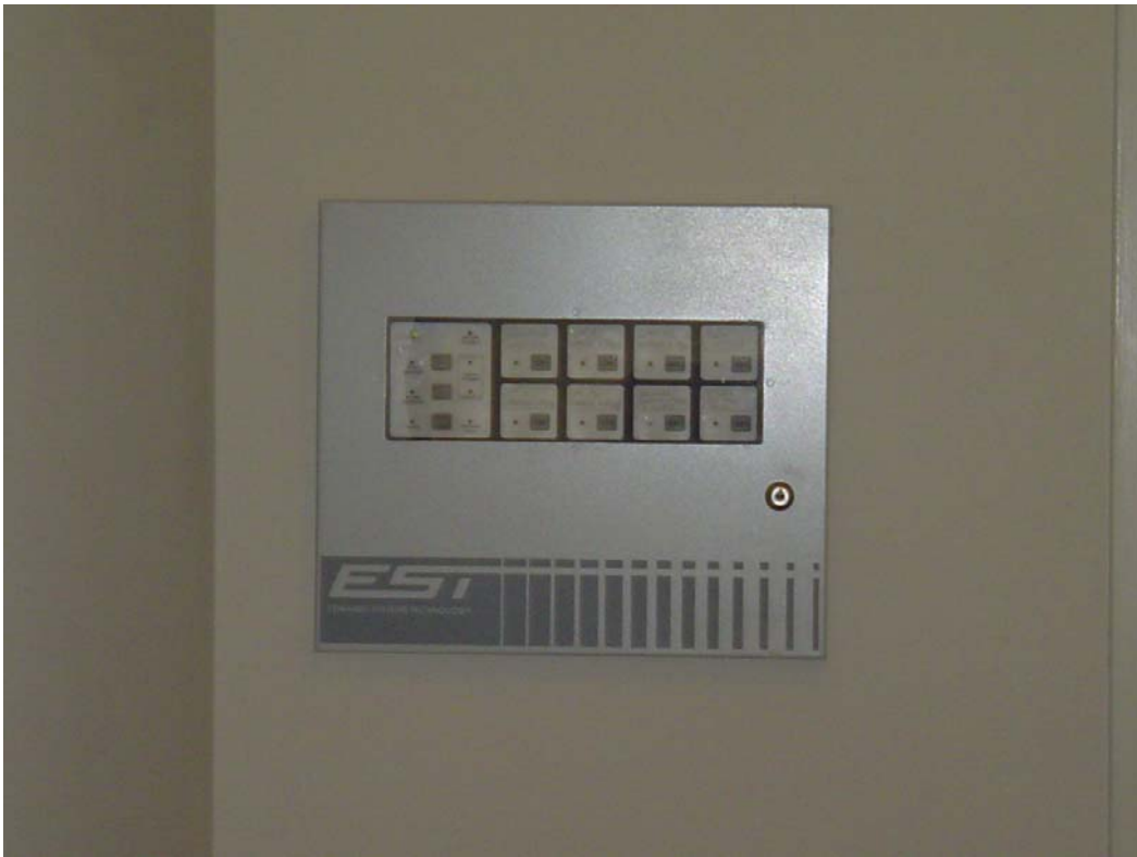
Typical Fire Alarm System Control Panel
